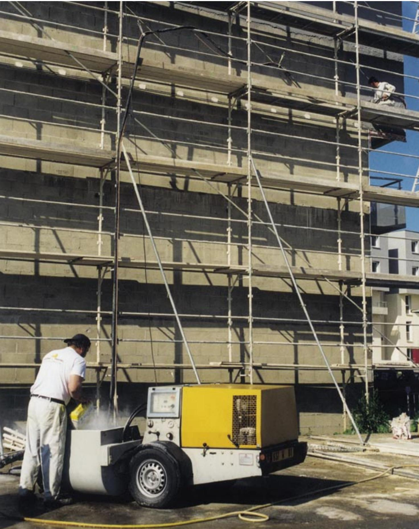
The SP 11 can also be operated by means of remote control from the spray gun so you do not have to depend on the machine operator.
